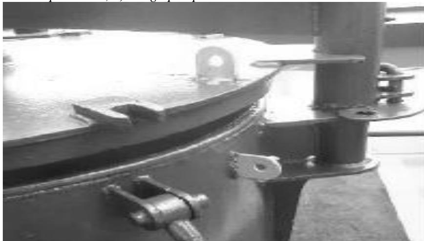
**Gambar 14.** *Manhole / Hatch Coaming*
